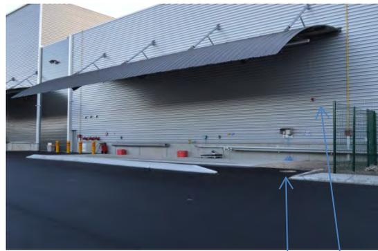
Chemical delivery area, note valve cover for drainage and sensors on wall
