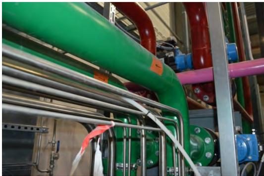
Showing colour coded pipework and welded joints ( Green = Polyol, MDI = Red, Octoate is pink)
