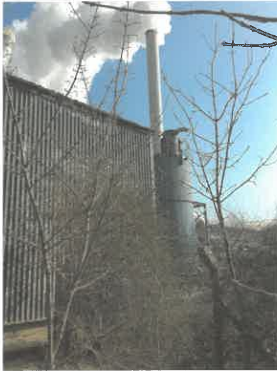
PHOTOGRAPH 1: S1 Dryer Plant Stack
