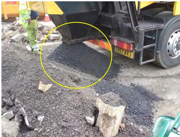
Fig. 4: Recycled material being deposited
